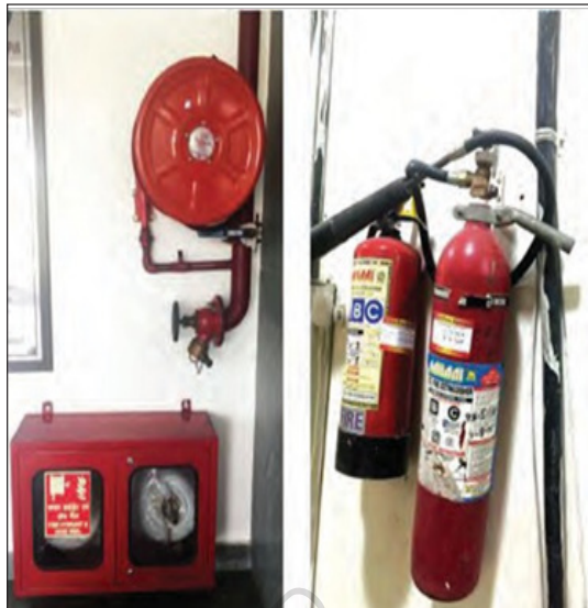
Fig.4.16 Fire extinguishers
